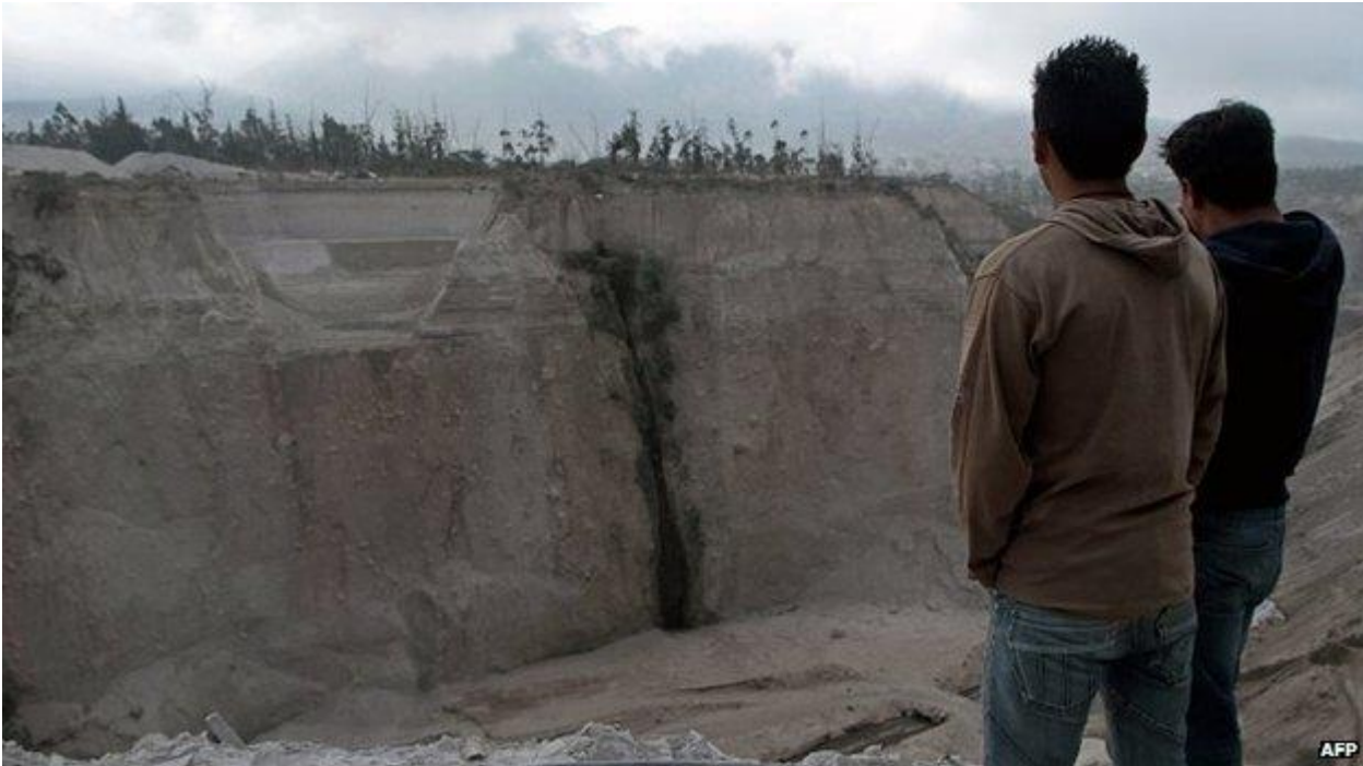
Four people are missing in the Catequilla quarry near Quito after the quake triggered a landslide
